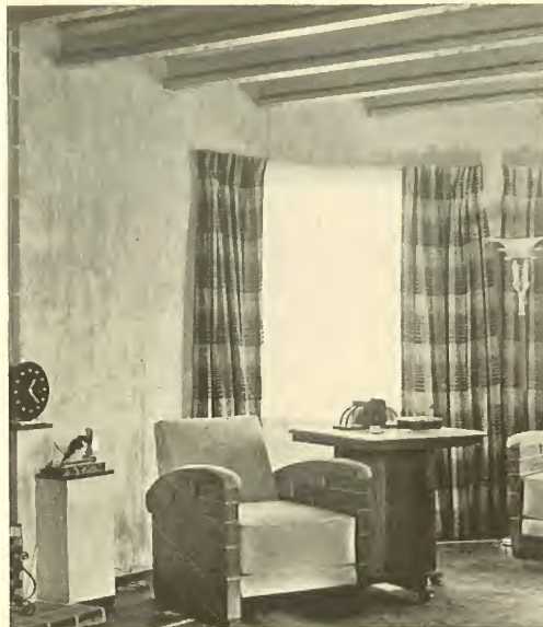
A living room corner in a concrete home in which the concrete floor joists become a lovely beamed ceiling.
